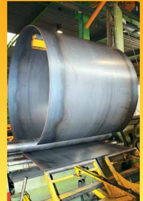
Tank rolling in progress
